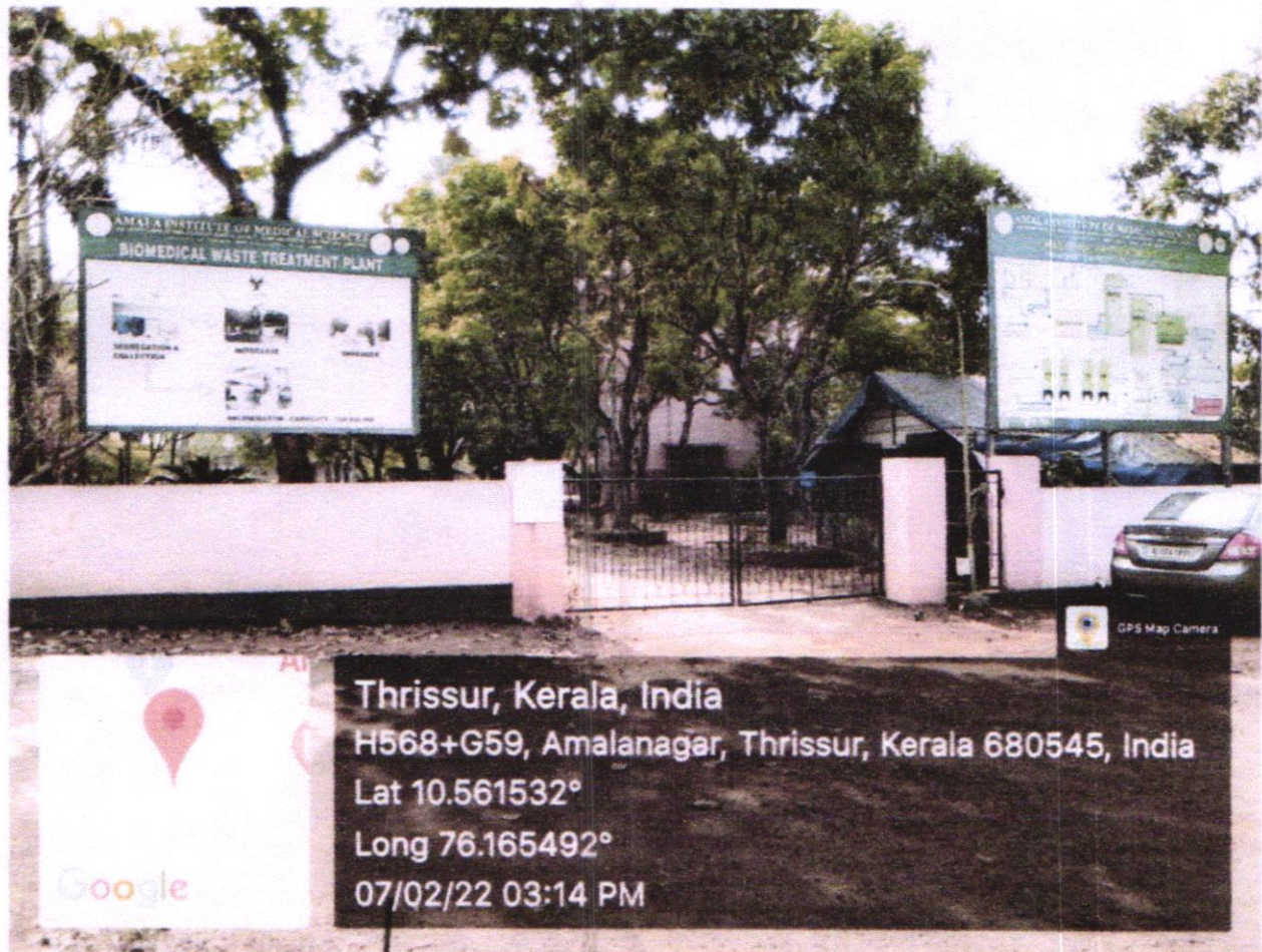
ACON, Waste water recycling plant and bio medical waste management plant
